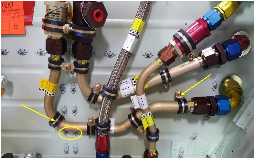
Figure 2. Tube assembly supporting clamps and possible fouling area.
