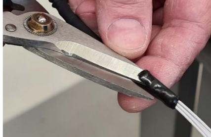
Figure 8 – Cutting the self-agglomerating silicone tape
